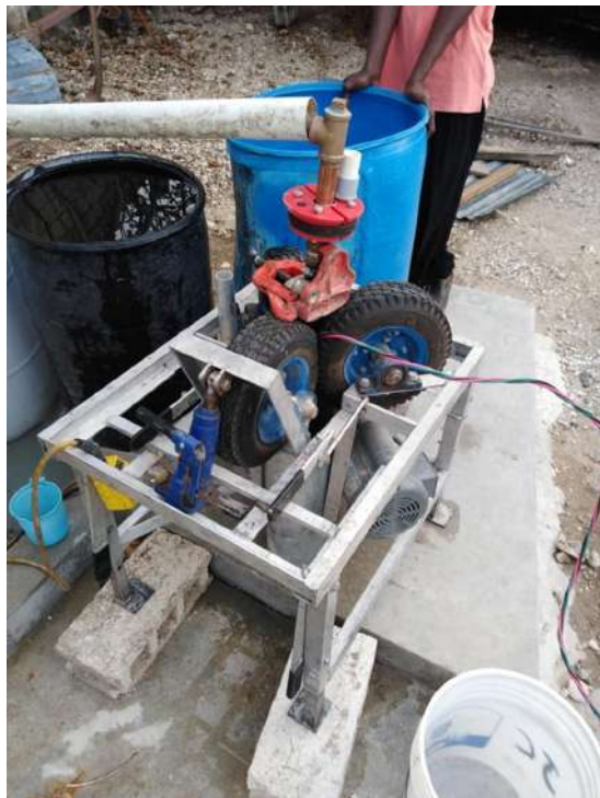
THE PUMP HAS BEEN INSTALLED
