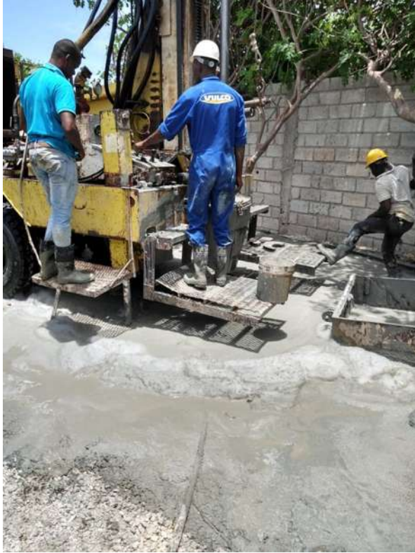
DRILLING THE WELL
